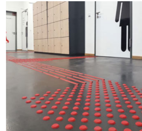
coloured tactile guidance system
