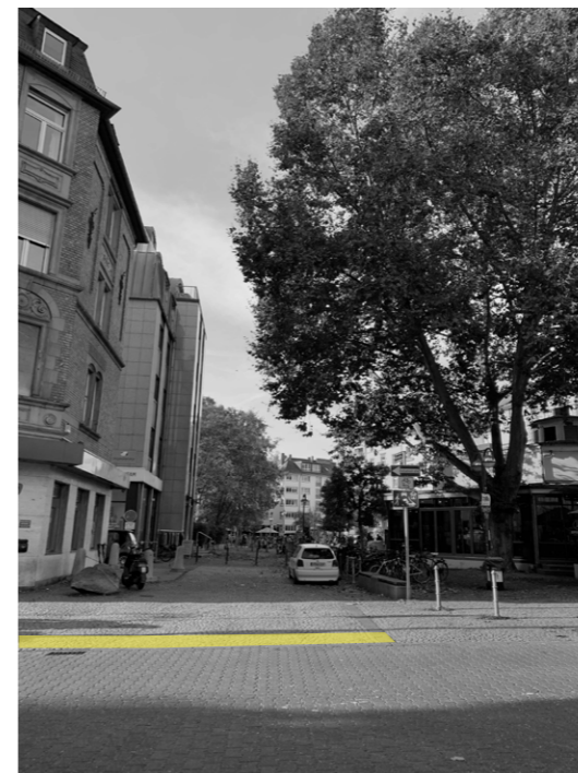
risk areas 4, 5, 6 there are two different fborings indicating crossing but no previous "warning" indicators
